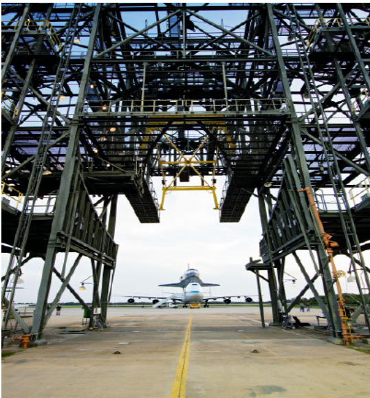
An orbiter atop an SCA is towed toward the MDD at the Shuttle Landing Facility at KSC. Once underneath the device, a hoist will lift the orbiter from the back of the SCA and place it on the ground.
